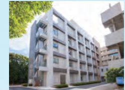
Yokohama City University Advanced Medical Research Center
