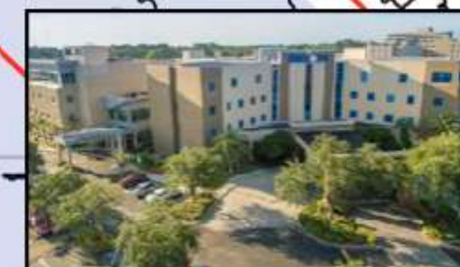
Brooks Rehabilitation (米国フロリダ州)
