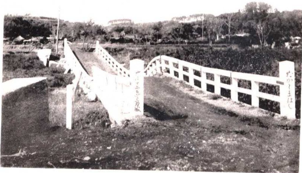
墜落せる縣道戸塚大船線高嶋橋
